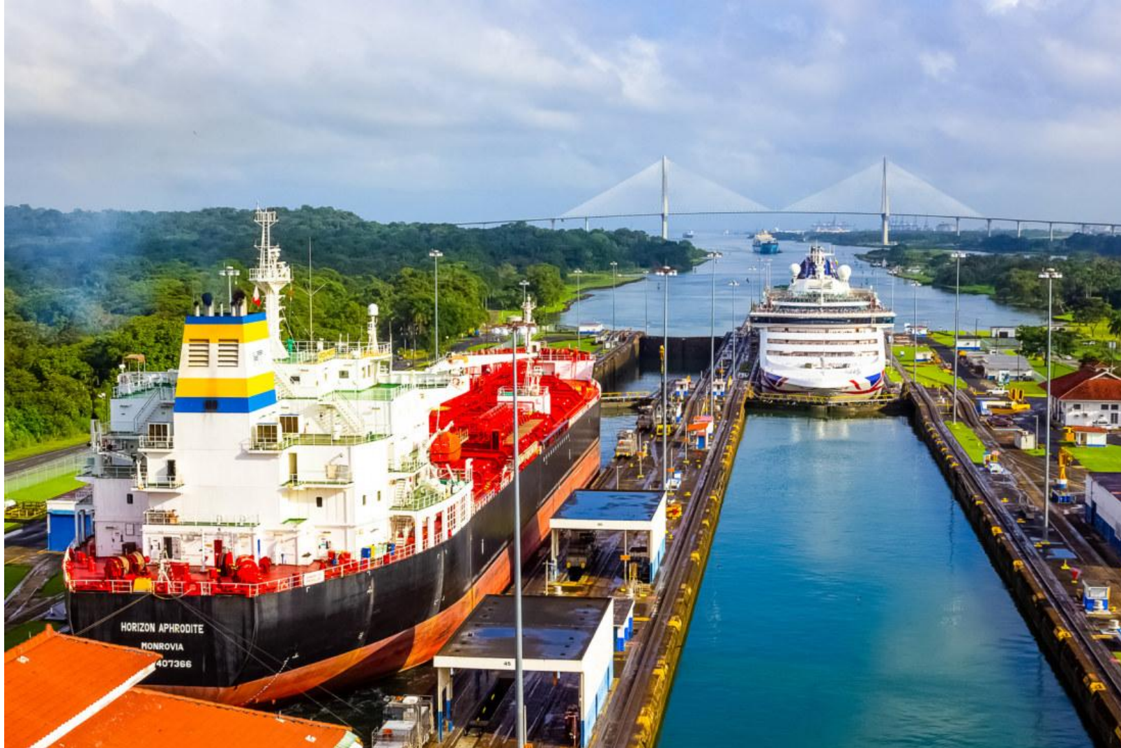
Entering from upstream into an empty lock
