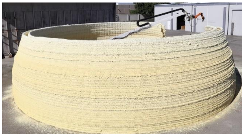
Figure 2 - Polyurethane insulation frame of a building
