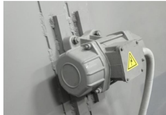
Figure 11 – Vibrator is installed on the hopper
